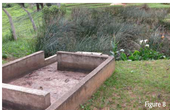
An example of a wastewater treatment system that was built in Rwanda to ensure compliance with Criterion 4.4 is shown in Figure 8.
